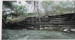
PILOT PROJECT BEFORE
