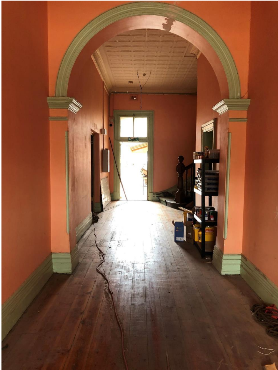
Ground Floor before the renovations
